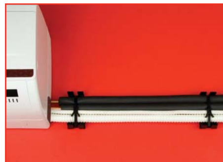
Lay the route and secure it using holders with tie
