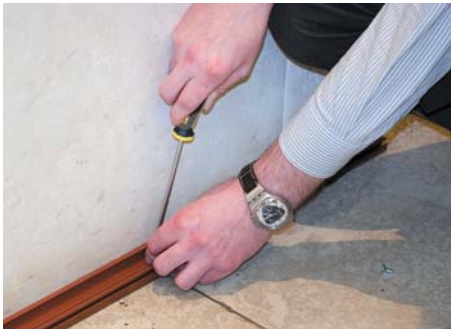
The duct base is attached to a floor, closely to a wall with lock outwards
