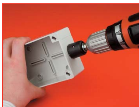
1 stage. Bore holes of required diameter
