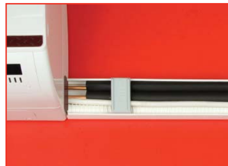
Secure the route in the duct base using attachment clamps
