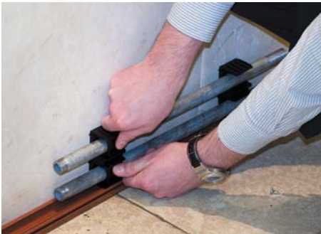
Universal holders are attached to a wall, closely to a duct base. The lines are attached in the holders
