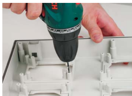
The socket is installed on new mounting seats. Since these holes are blocked from the front by default, through-holes shall be made with a drill bit 3 mm for ease of installation. Holes are not required if socket with flange 70x87 mm is installed, for example, DIS5706407
