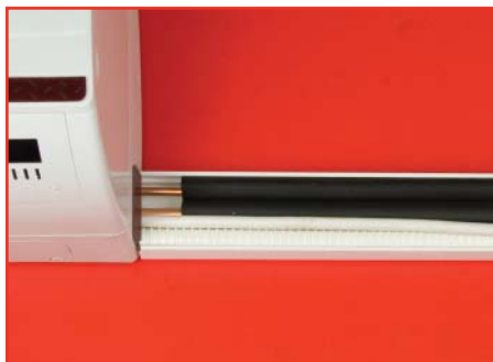
Lay the route in the duct base
